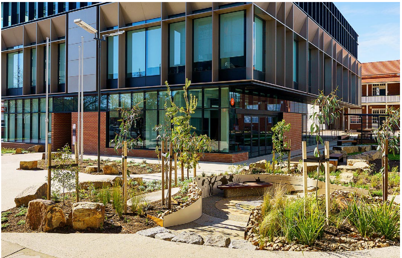
The Djjimbayang Indigenous Engagement Centre in Building J at Bendigo City campus.
